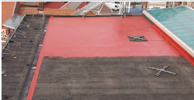
During: Application of Sika Decothane Waterproofing System
