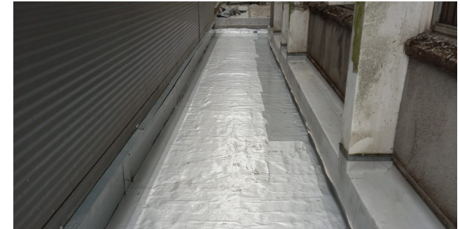
During: Insulation and VCL Installed on Gym Walkway
