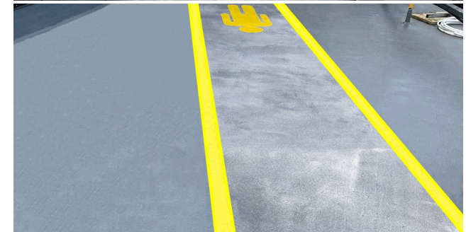
After: Vibrant New Line Markings on Gym Walkway
