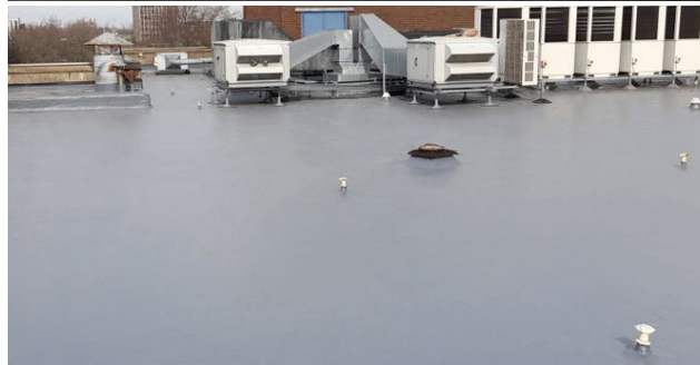
After: Fully Re-Waterproofed Roof Area
