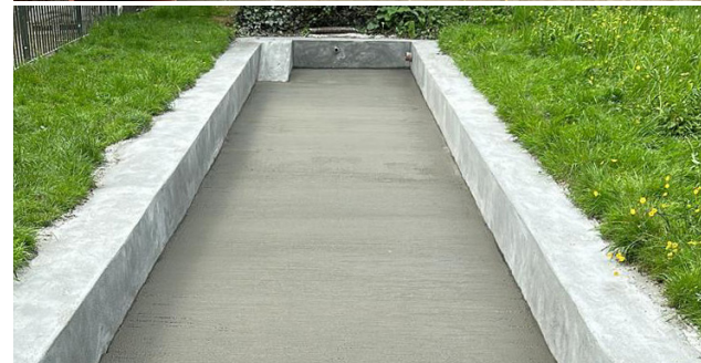
After: Completed Waterproofing
