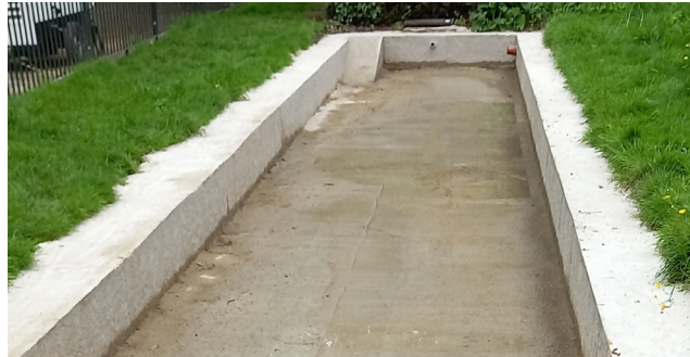
Before: Re-cast Concrete Ready For Waterproofing
