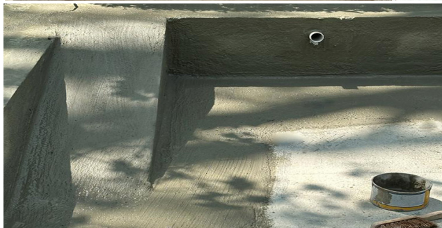
During: Waterproofing To The Walls & Floor
