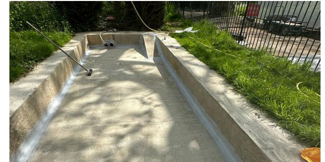
During: Application Of Sikadur Combiflex
