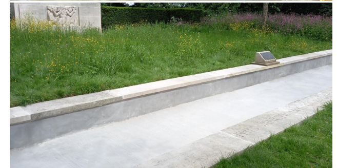
After: Sealed & Watertight Pond
