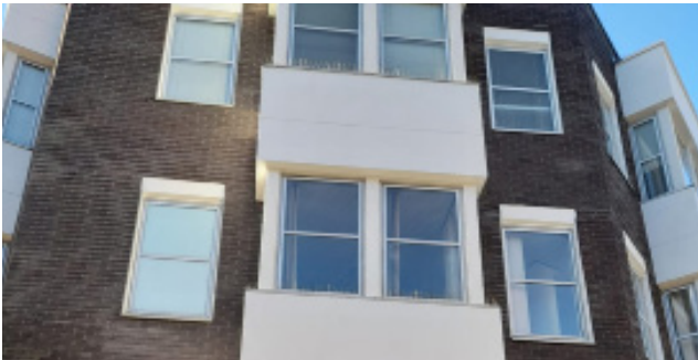
After: Repaired & Renewed Facade
