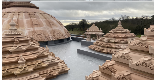
After: Fully Protected Warm Roof
