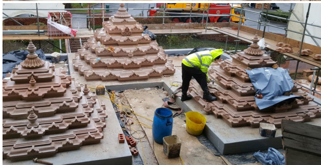
During: Reinstatement of Stone Structures
