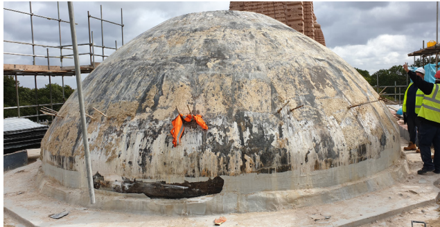
During: Removal Of Existing Waterproofing System
