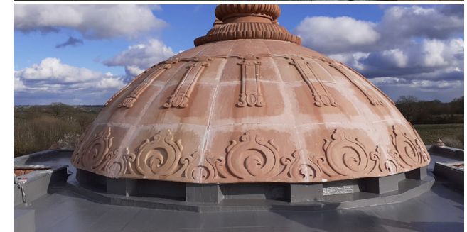
After: Waterproofing Temple Roof & Dome
