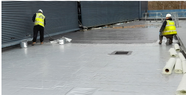
During: Application of Low Odour Waterproofing System
