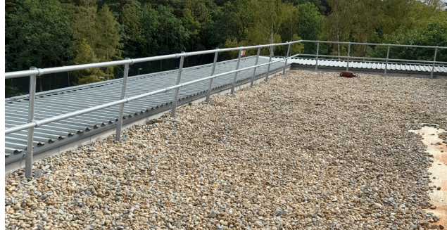
Before: Pebble Ballast & Cracked Asphalt
