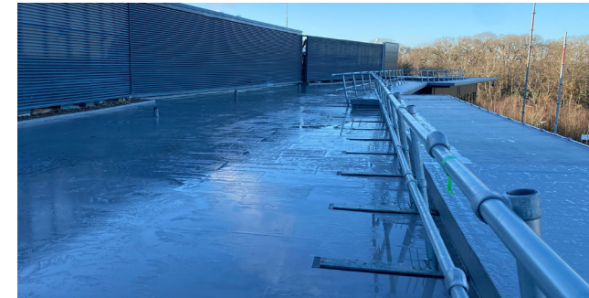
After: Fully Watertight With No Ponding Issues
