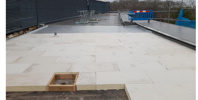
During: 120mm Thick Insulation and VCL
