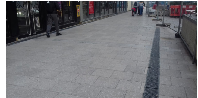
After: Watertight & Drainage Issues Resolved
