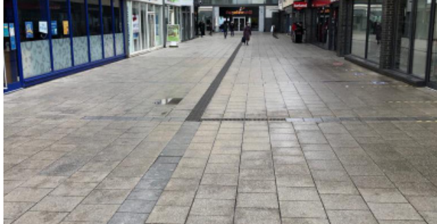
Before: Podium Deck With Water Ingress Into Train Platform Below
