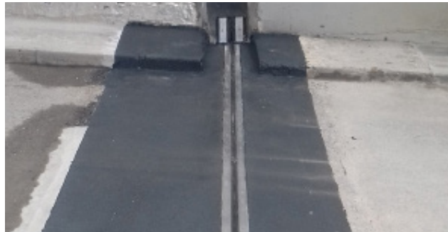
During: New & Bespoke Movement Joints
