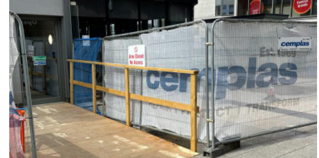
During: Temporary Ramps & Walkways
