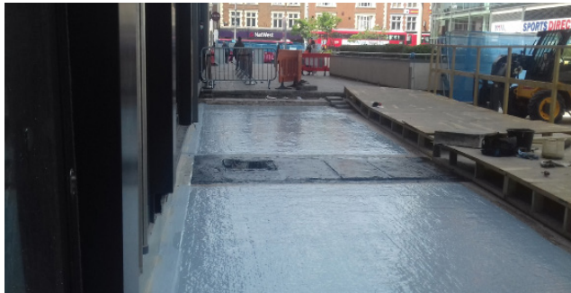
During: Podium Deck Waterproofing Membrane
