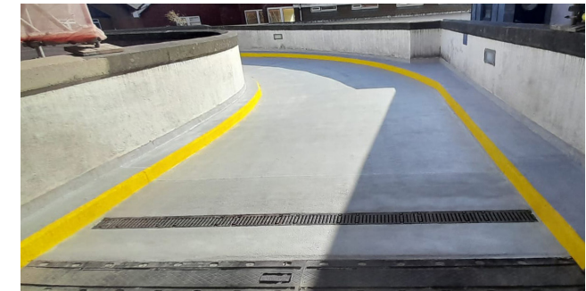
After: Replacement Expansion Joint
