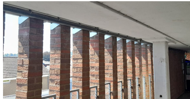
After: Light & Bright Interior Improvements
