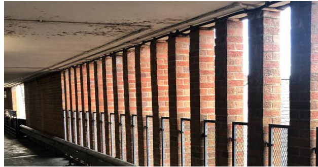
Before: Decks & Columns Unprotected
