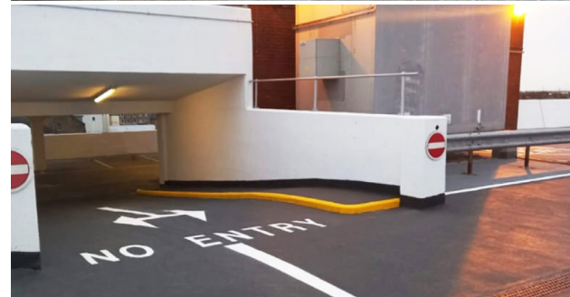
After: Fully Protected Decks & Columns
