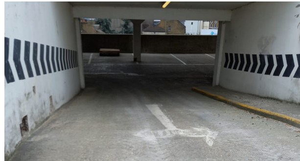
Before: Decks & Columns Unprotected
