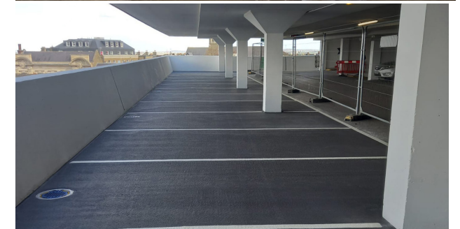
After: Perimeters Waterproofed With New Drainage Channels
