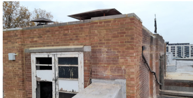
After: Fully Protected Steelwork & Reinstated Brickwork
