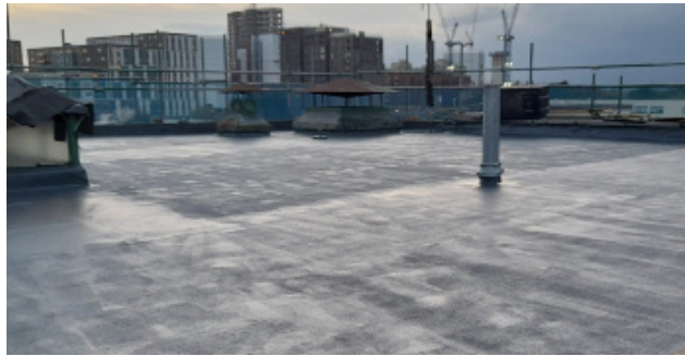
After: Watertight Overlay of Roof
