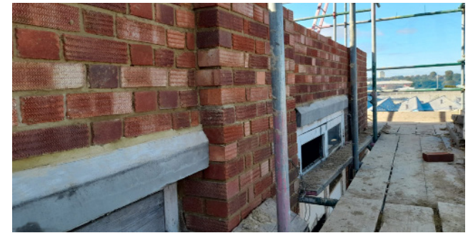
After: Repaired Cills & Brickwork
