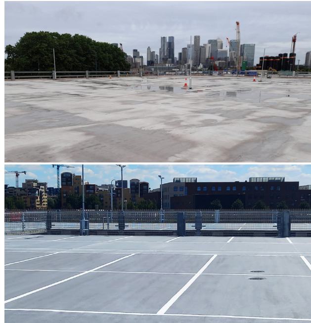
After: Fully Protected & Watertight Decks
