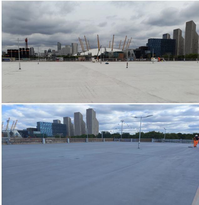
During: Installation of Deckshield Rapide ED1
