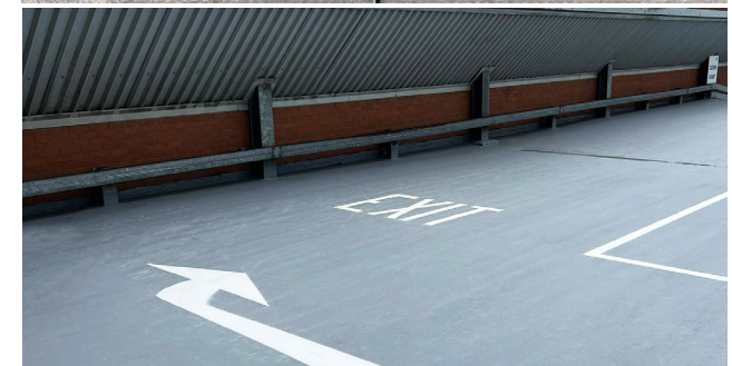
After: Application Of New Line Markings
