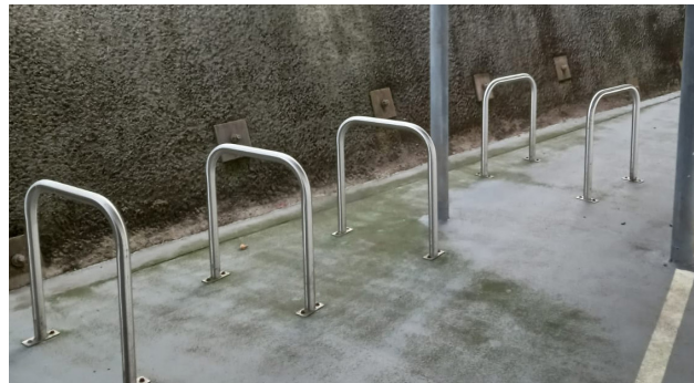
Before: Cliff Edge & Car Park Connected
