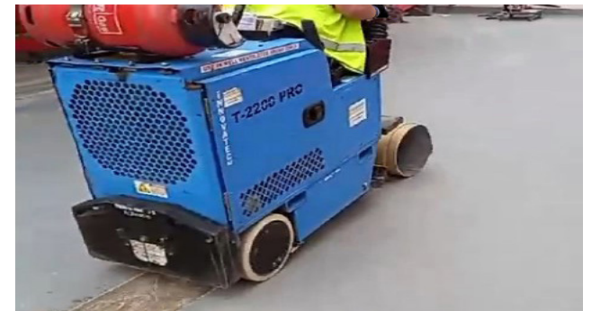
During: Coating Removal With Weight Restrictions
