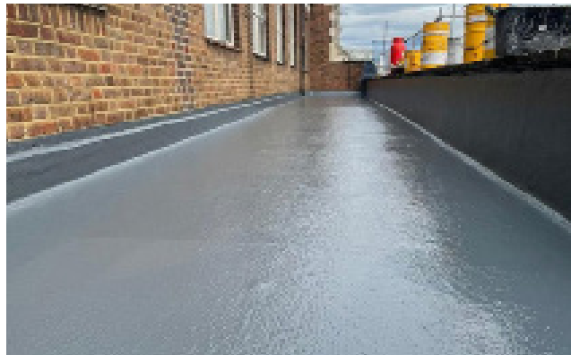
After: Thermally Upgraded & Watertight Walkway
