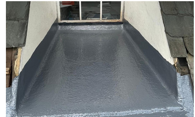
After: Waterproof Detailing Expertly Carried Out
