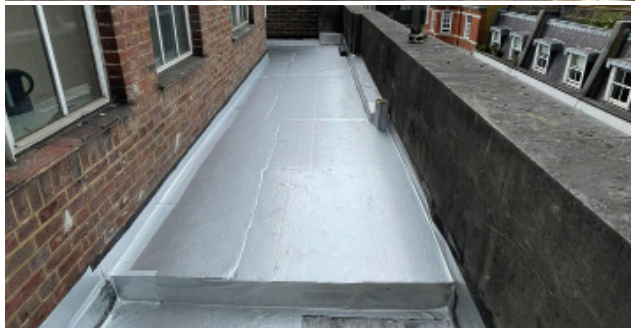
During: Installation Of Insulation & VCL
