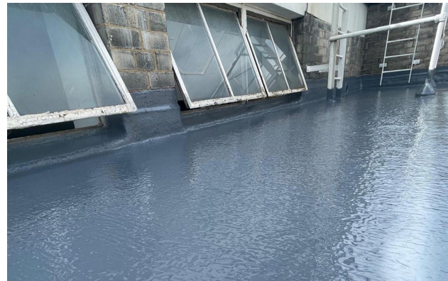
After: Fully Re-Waterproofed Roof Areas
