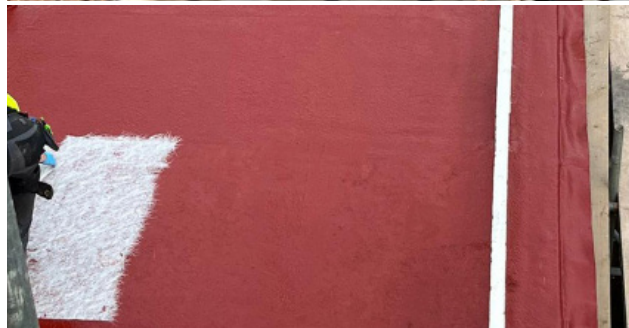
During: Application Of Reinforcement Fleece with Primer
