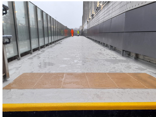
After: Walkways Enhanced & Upgraded
