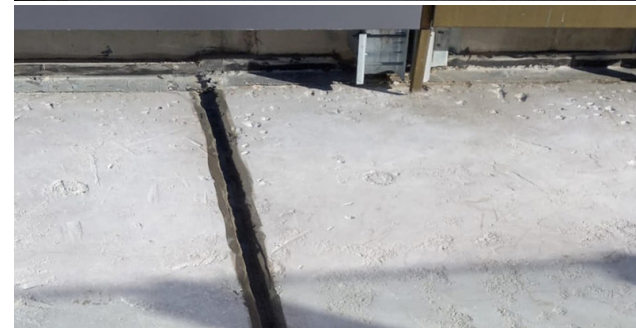
During: Widening Of The Expansion Joints From 10mm to 30mm
