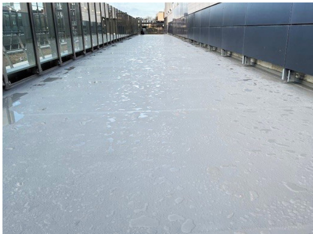
During: Watertight Walkways
