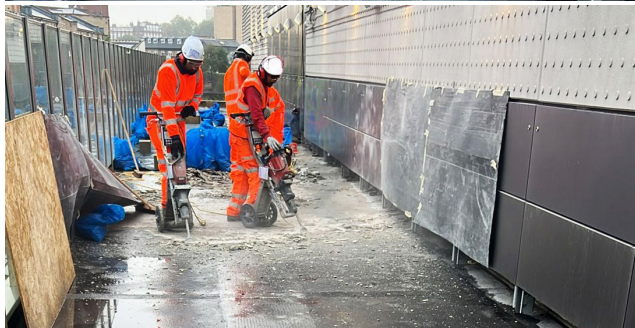
During: Removal Of The Existing Waterproofing System
