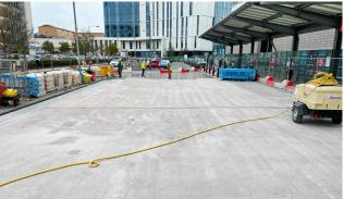
adhesion of the Sika RB28 resin, a vital component of the waterproofing solution used.
