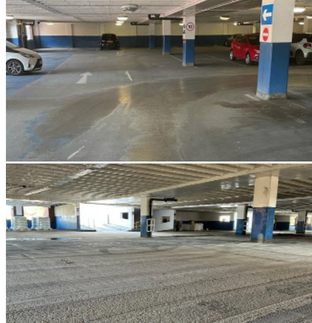
During: Concrete Repairs Completed and Decks Prepared
