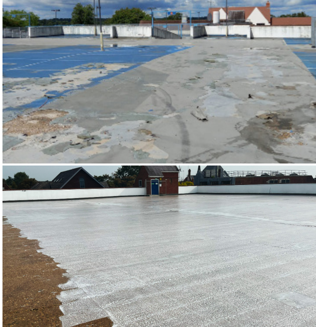
During: Pre-Primer To Combat Outgassing
