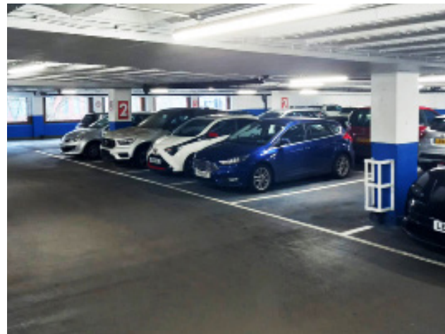
After: Light & Bright Interior Improvements
