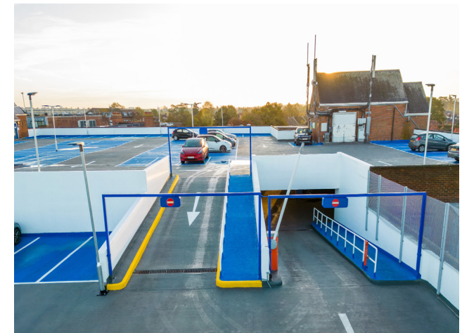
After: Fully Protected Decks & Ramps
