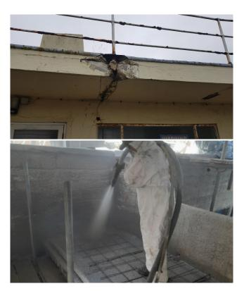
interventions to restore the building's integrity. A key element was implementing corrosion protection techniques, such as cathodic protection, which stops corrosion to the rebar within the concrete. Highperformance repair mortars complemented these methods, restoring the structural integrity whilst respecting its historic aesthetic.
