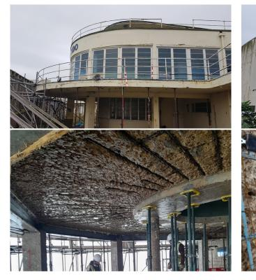
Saltdean Lido, a Grade II listed building, is a rare example of Modernist seaside architecture, renowned for its Art Deco style and distinctive ship-like façade. Constructed using reinforced concrete with slim walls and minimal structural supports – a groundbreaking feat at the time – its unique features have earned it a celebrated status. English Heritage recognised the Lido as one of the 'Seven Wonders of the English Seaside', further cementing its importance as a historical landmark.
