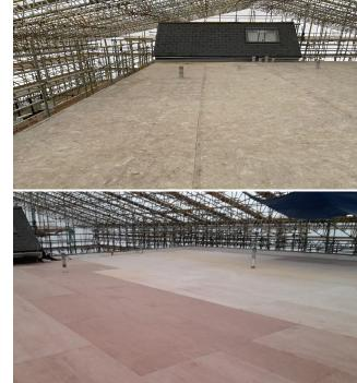
St Georges Court is a multi-storey residential building which faced significant issues with its waterproofing and insulation systems. The single ply membrane on the main roof and the liquid-applied coating to the terraces had deteriorated, leading to water ingress and potential damage to the underlying timber deck.
