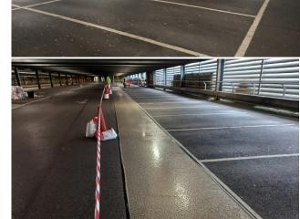
The MSCP at Queens Hospital in Romford recently underwent a refurbishment to address the worsening condition of it's asphalt top deck, which had reached the end of it's lifespan. Over time, wear and tear had led to visible defects such as wheel indentations, potholes and general asphalt breakdown.
