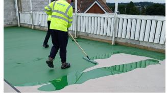
The first visible issues arose on the top decks, where the original waterproofing system had reached the end of its serviceable life and was delaminating from the substrate. Without this protective layer, the concrete became increasingly vulnerable to persistent water ingress.
