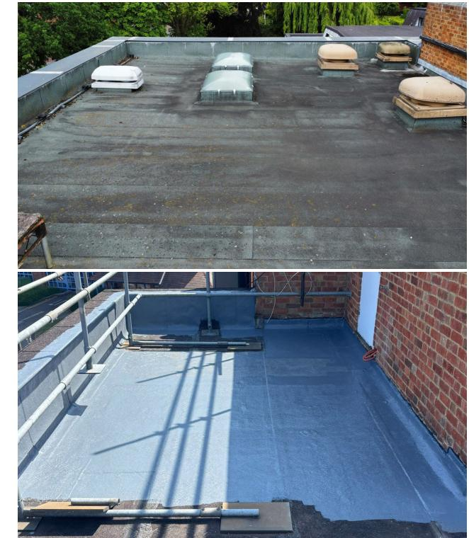
continuous waterproofing termination that integrated seamlessly with the existing roof structure.
