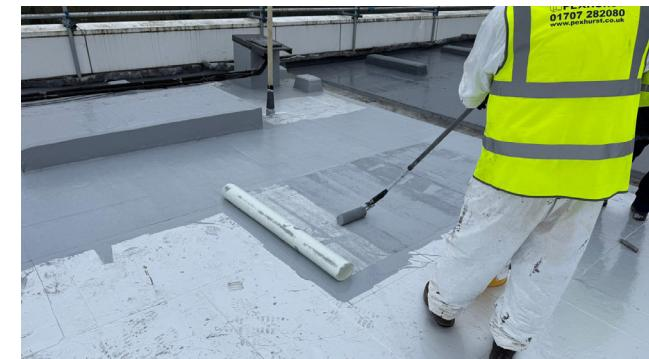
**Elder House is a well-known office building in the center of Milton Keynes, providing workspace and meeting facilities for a variety of businesses. The building's existing roof waterproofing system had reached the end of its serviceable life after years of exposure and patch repairs. This deterioration prompted the application of a durable, thermally efficient and fully waterproof replacement.**
